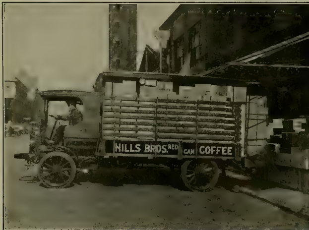
Model 27K, 4-cylinder Autocar. 138 inch wheelbase. 2-3 ton with overall carrying capacity of 15,000 pounds, turning circle 45 feet.
